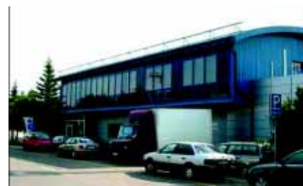
External view of the cargo terminal.
